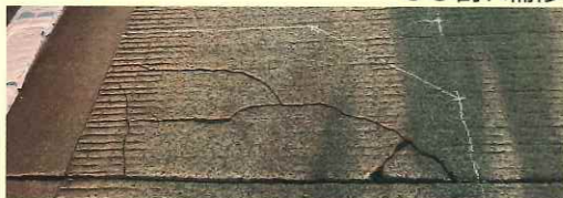
ひび割れ補修
